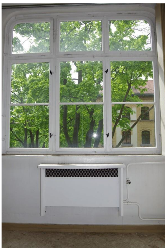
Veranda Detail Fenster
